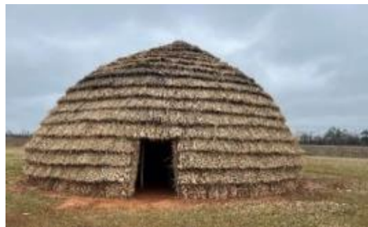
Figure 4. Caddo Indians use switchgrass to build houses and ceremonial structures. Photo by ETPMC.
